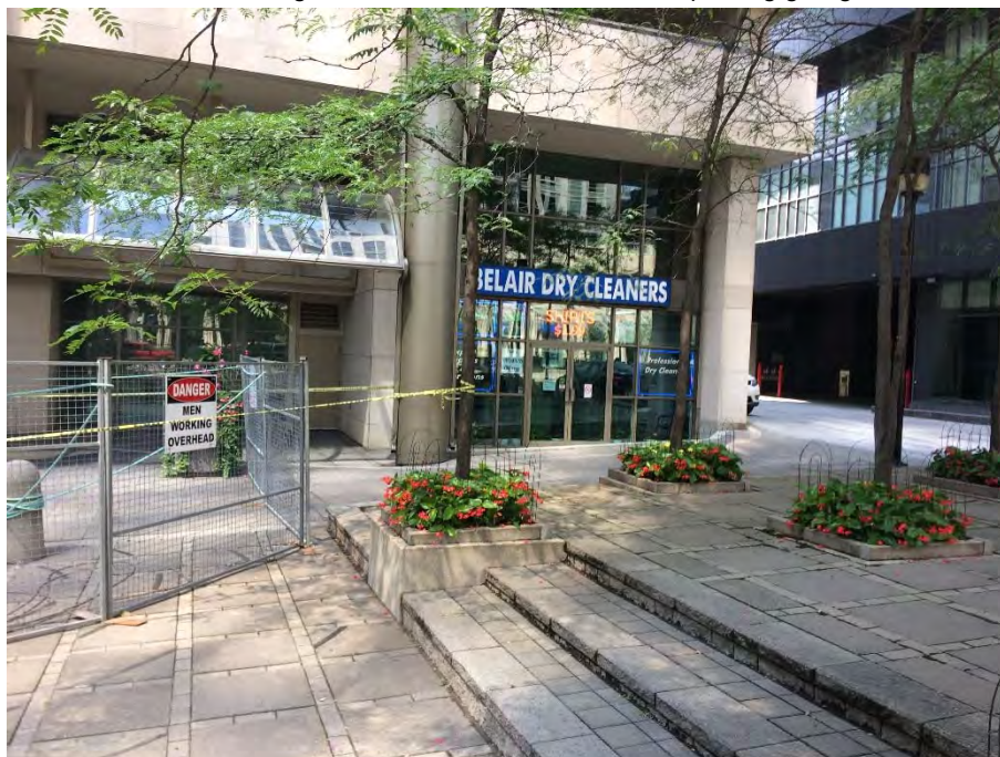
Photograph 14: Dry cleaning depot at neighbouring 750 Bay Street, to the west of the Site, facing west. Located at the first floor of a multi-storey residential condominium
