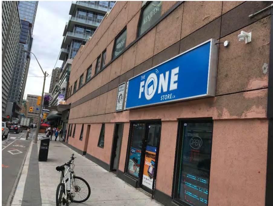
Photograph 21: Typical store fronts, offices and residential buildings at the corner of Yonge and Gerrard Street, facing west from Gerrard Street E towards Yonge St.
