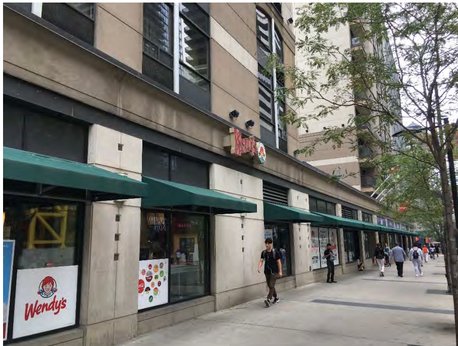
Photograph 16: Typical store fronts and offices along Yonge Street south of Alexandra Street, facing southeast towards Wood St.
